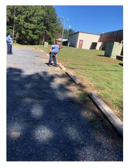
The front wall of Building 500 has some water issues. Upon investigation, it was found that the front foundation seal is failing. To repair this, the maintenance crew will dig along the brick portion of the wall (grassed area), install drainage pipe along edge, and back-fill with gravel. The stucco walls along the front sidewalk also requires repairs.
