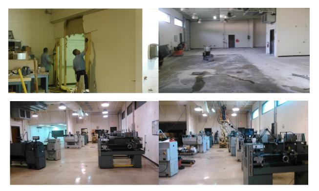
The wall between Rooms 507 & 508 has been removed to accommodate the lecture and physical training for Department of Correction employees. After the wall was removed, carpet was removed, the concrete floor ground, dyed, and polished.
