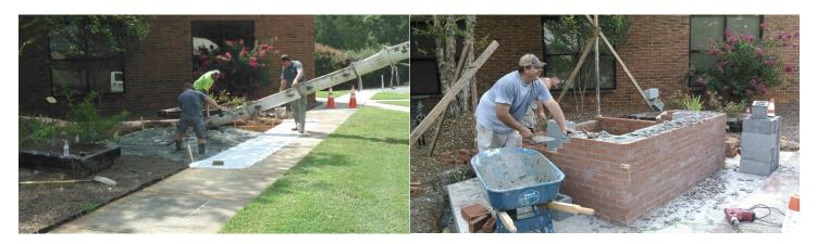
The MCC Bell project is underway with the pouring of the foundation and building of the support structure. We are looking to have the bell finished before the September  $7^{th}$  ceremony.
